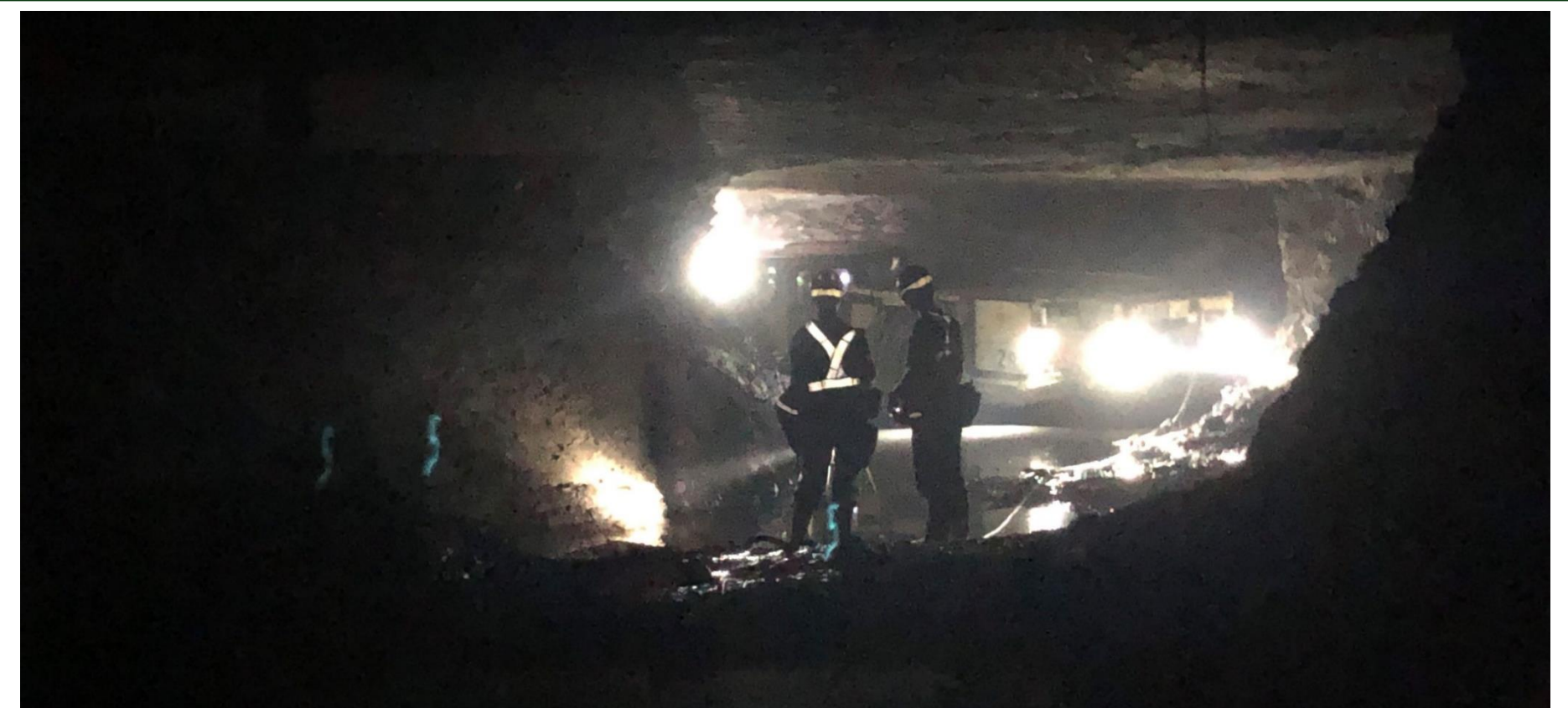
Figure 1. Excavation of an underground mine
